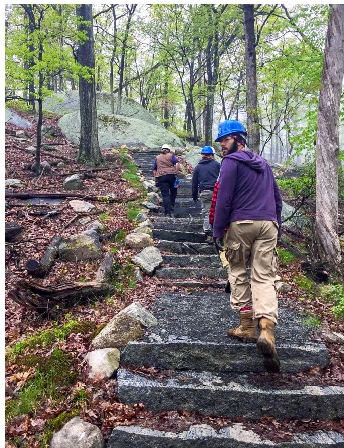
More than 1,300 stone steps were placed on Bear Mountain to make the Trail here sustainable.
